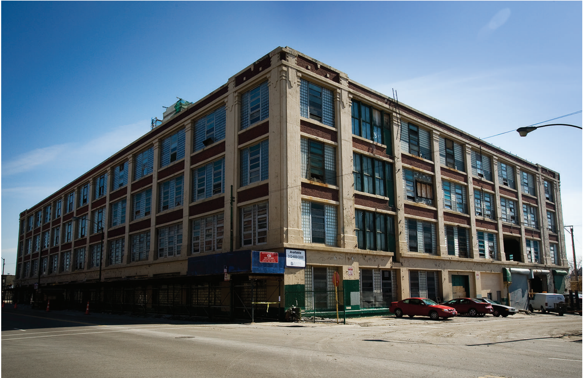
The old Frederick Cooper Lamp Company, 2545 W. Diversey Ave., is slated to become the Green Exchange building, the first green mall in the Midwest according to leasing director Phil Baugh.
