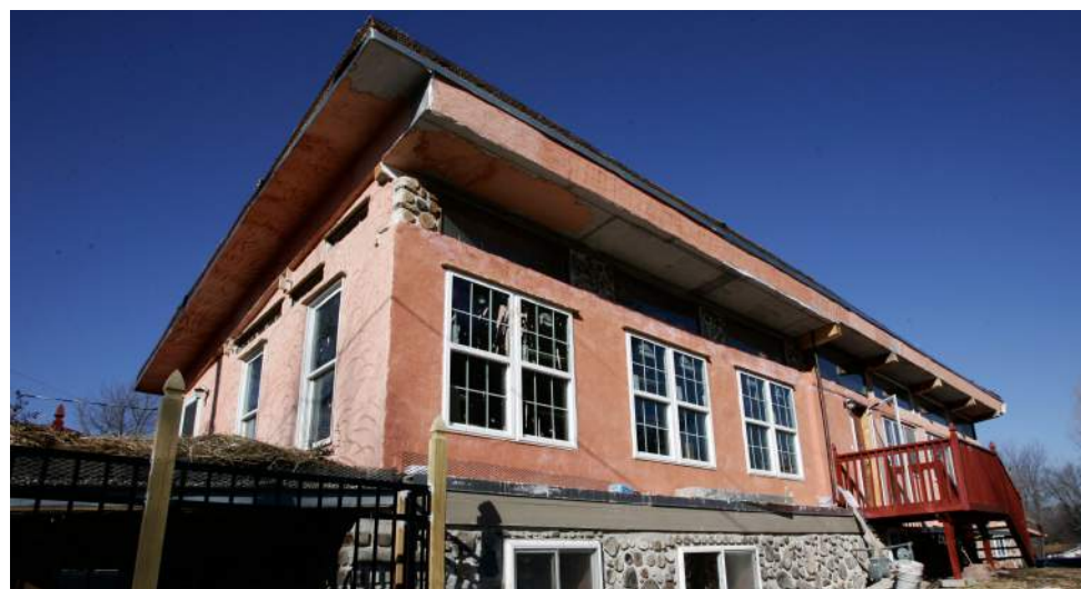
The hybrid home of John Schulz is being built with straw-bale walls, cord-wood masonry, passive solar heating, a natural stone retaining wall, an earth-sheltered lower level, no air conditioning and an insulated, zero-maintenance green roof that could last 80 years with five inches of soil, flowers and shrubs growing on top of it.
