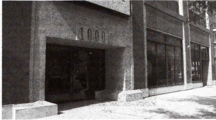
Columbia purchased 1000 S. Wabash Ave., above, and 916 S. Wabash Ave., from the Chicago Housing Authority in July. Construction should begin by spring 2008.
