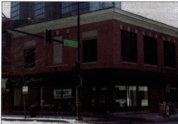
On the corner of Balbo and Wabash Avenue, the new Kinko's undergoes construction.
