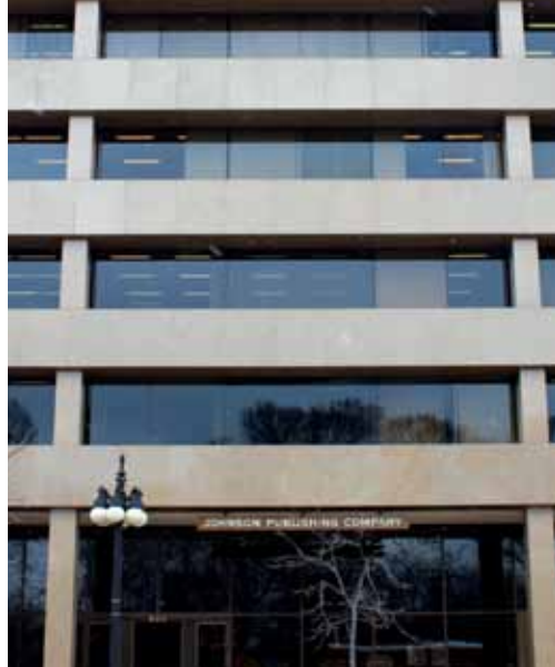
The campaign is raising funds for capital projects. The Averill and Bernard Leviton A+D Gallery at 619 S. Wabash Ave., which showcases student and professional works, needs to be refurbished. Columbia acquired the Johnson Publishing Company building at 820 S. Michigan Ave., historic home of Ebony and Jet magazines, in 2010. The building will house the college's ever-expanding library. Photos: Latrice Dixon
