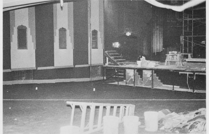
Eleventh Street Theater renovation (in progress).
